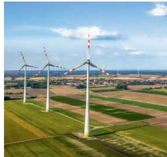
VIG is supporting the transition to renewable energies, for instance by insuring stations for wind power and other green energies.
