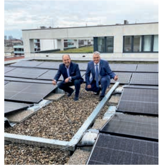
A photovoltaic system generates environmentally friendly electricity on the roof of the Linz location of Wiener Städtische and Donau Versicherung.
